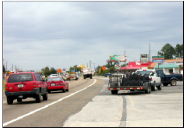
Undefined Driveway Affecting Driver Expectancy
