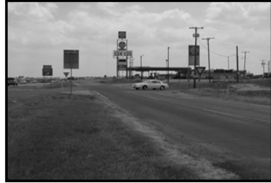
Unsafe Weaving Conditions
